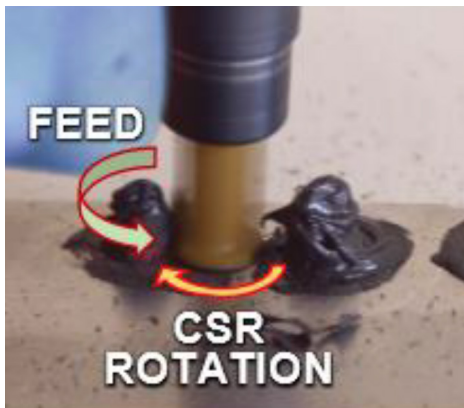
BA 4115 fastener sealant removal
