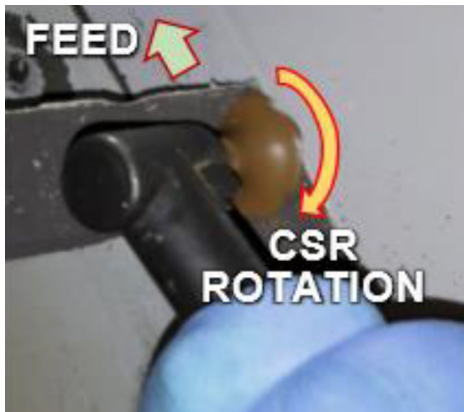
BA 4110 general sealant removal
